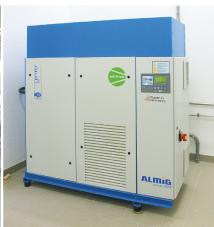
03 Prolupin, based in Grimmen, northern Germany, generates the compressed air needed for various stages of production with a compressing Lento screw compressor which is absolutely oil-free right from the outset
